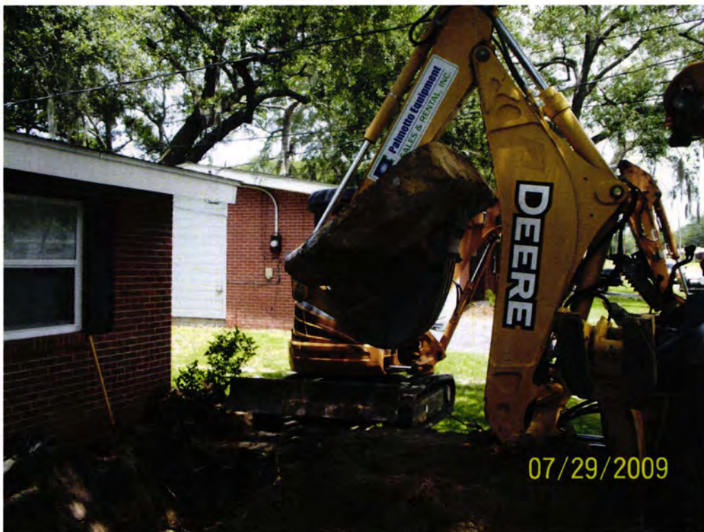
Picture 2: Removal of Concrete cover over UST 1411 Eagle-1
